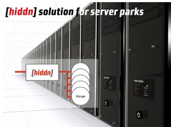
Figure 14 [hiddn]™ Serverpark Application
